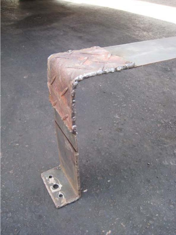
Repaired and reinforced bracket.
