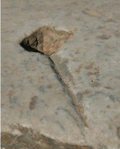
A junction between two sections of a marble column. The sections were joined by short pieces of iron and molten lead was poured down the channels to lock the iron in place. This method of construction was extremely vulnerable to earthquakes, which destroyed most ancient cities in this region. Ancient Ephesus, Turkey.
