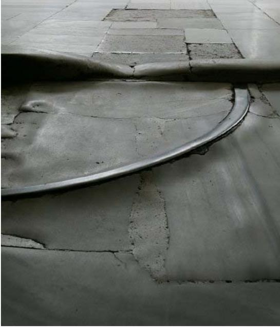
Worn marble doorway at Topkapi Palace. The metal track is for a roller on the bottom of the door. The palace was built in 1457. Istanbul, Turkey.
