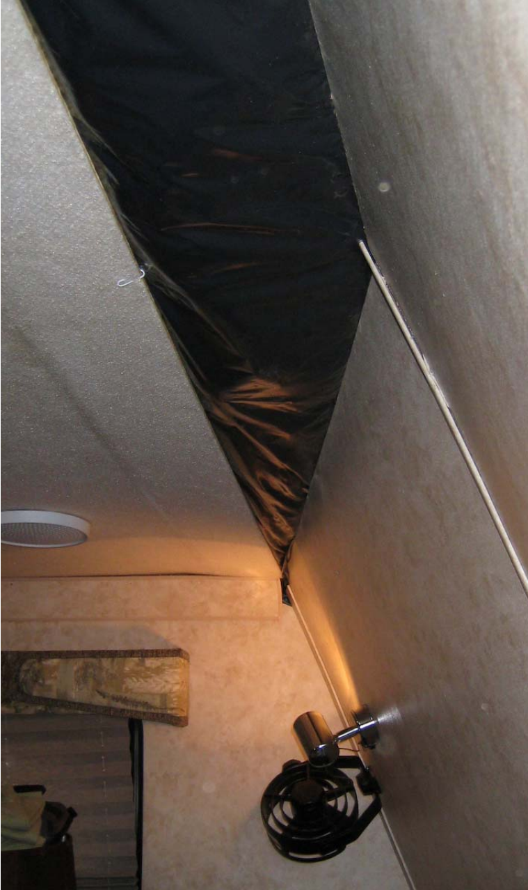
Moisture barrier extends from bulkhead and is tucked behind forward wall panel.
