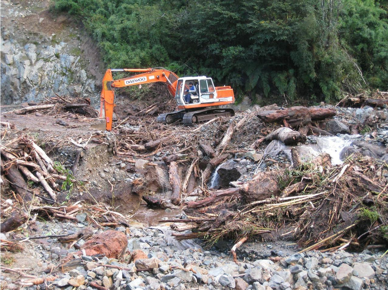
The hoe working on unplugging the bridge. The bypass river channel cut by the flood waters is in the foreground.
