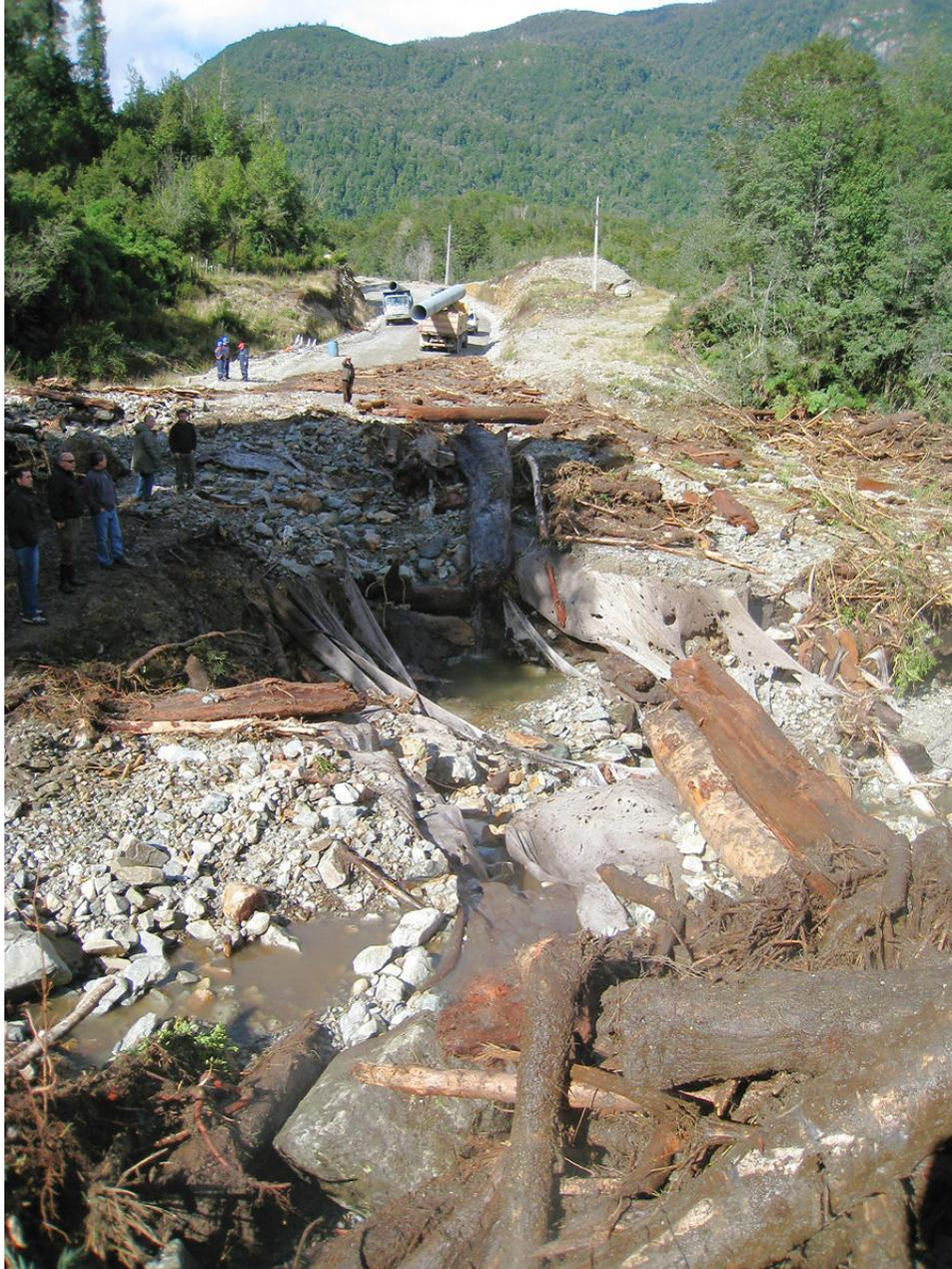
The view looking back up the road we were parked on. The bypass channel cut by the flood waters is in the foreground. Note the road bed fabric liner. The road that was destroyed was a very new road.
