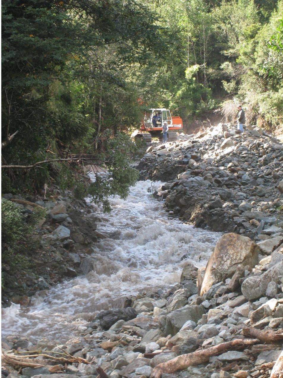
This is the view looking up the normal, original course of the river. The hoe is working to build up the banks to seal off the bypass flood channel created in the storm. The hoe created a path for itself all the way up the river and re-created this original, normal river channel.
