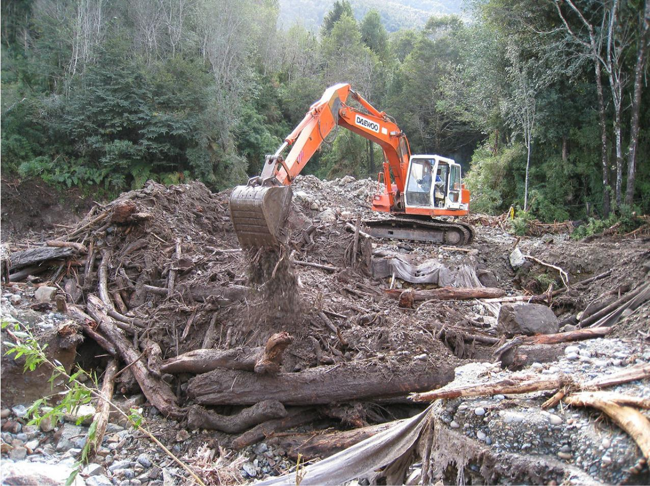
The hoe building the temporary bypass road. Note the size of the debris and boulders.
