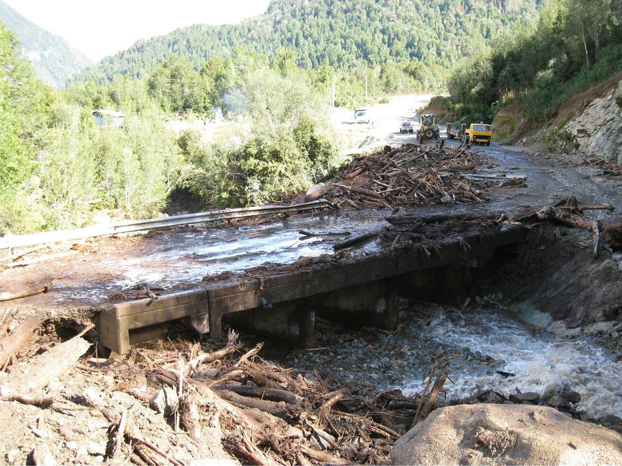
A view of the bridge after the debris that plugged it had been cleared. Note the debris piled on the far side of the bridge.
