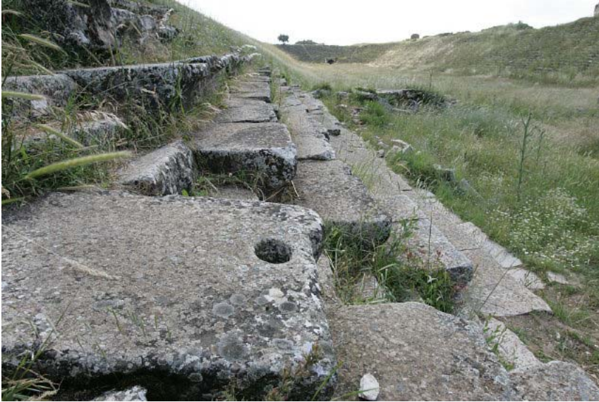
Seat detail at the stadium. The hole is not a cup holder; it was used to hold up a stanchion supporting an awning to shade the crowd from the sun. There were reserved seats in the stadium, which were carved with the owner's name. Ancient Aphrodisias, Turkey.
