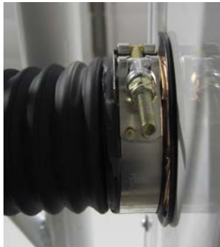
Waste water input to macerator pump
