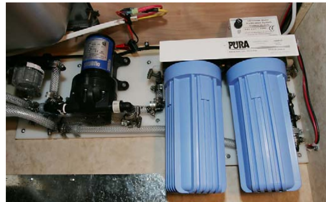
Fresh water transfer pump and UV filter assembly
