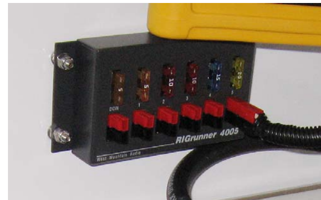
Shop 12VDC fused outlets
