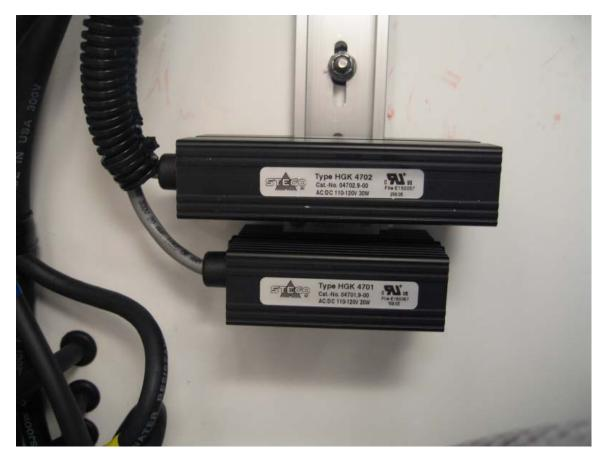
You're probably thinking the same thing I was, "50 watts! How can you heat a box that big with only 50 watts?" That's how I ended up with 50. I started with the 20 watt unit and ordered the additional 30 when I couldn't sleep at night.
