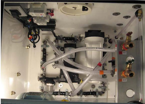
That yielded a raw water compartment that can keep itself warm and the water, hoses, pump, filter, etc. from freezing (hopefully!)
