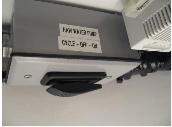
First, the switch that controls the raw water pump in a weatherproof box with a waterproof switch.
