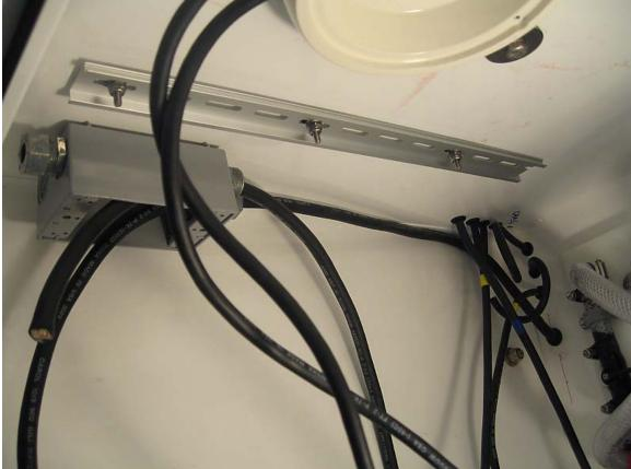
First, I test mounted the DIN rail that everything attaches to.
