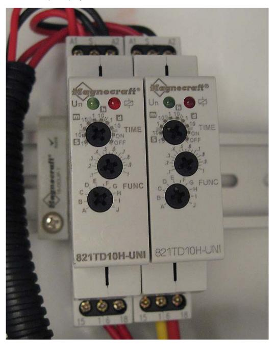
Just to keep things interesting, Magnecraft changed the function program definitions between the time the one on the left was built and the one on the right was delivered, so I had to interpret two different sets of functions and profiles to get this set up.
