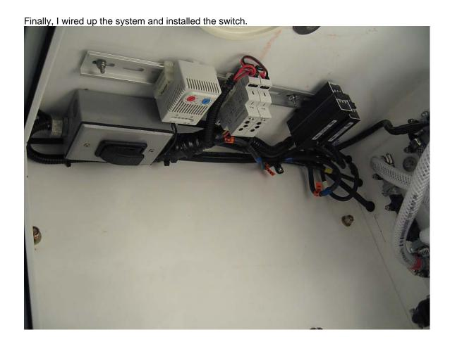
That yielded a raw water compartment that can keep itself warm and the water, hoses, pump, filter, etc. from freezing (hopefully!)
